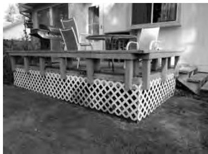
Rot and mildew were just two of the problems the old deck posed the homeowners.
